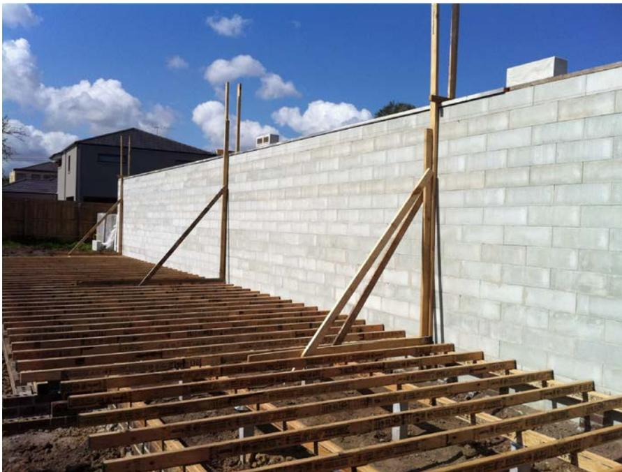
Benex Block walls with returns should be checked for lateral stability. As a rough guide, if a return on a wall is less than 600mm then that end of the wall is without adequate lateral support and requires fixing to a support or bracing.
